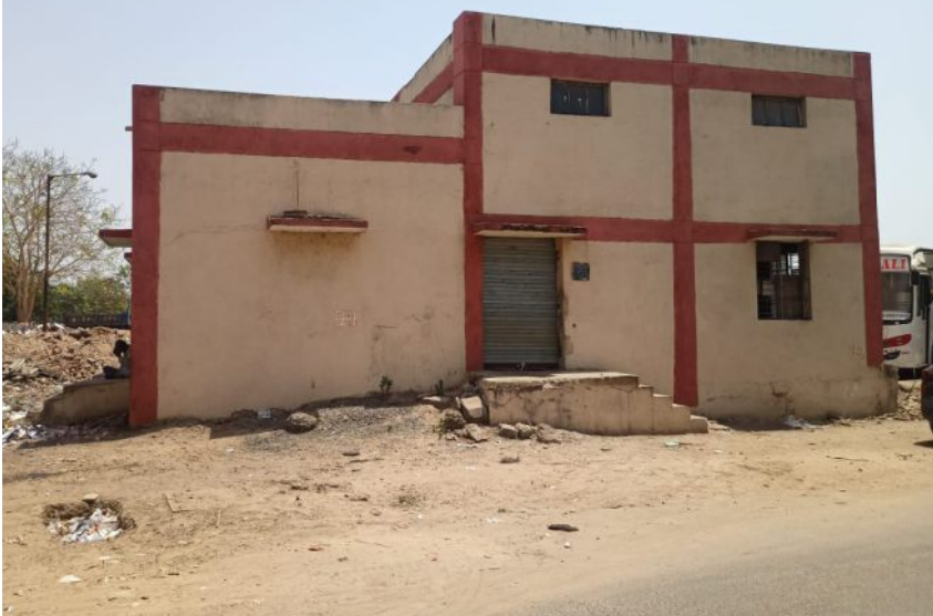
Sureliya SWD Pumping Station
